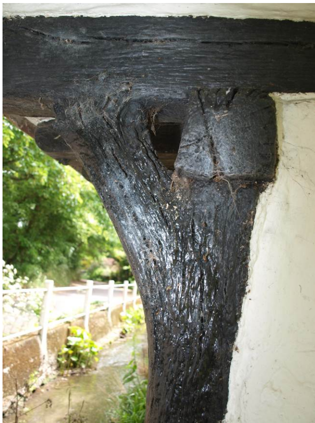
Plate 2: Naturally forked timber for post and brace under north end jetty west side)
