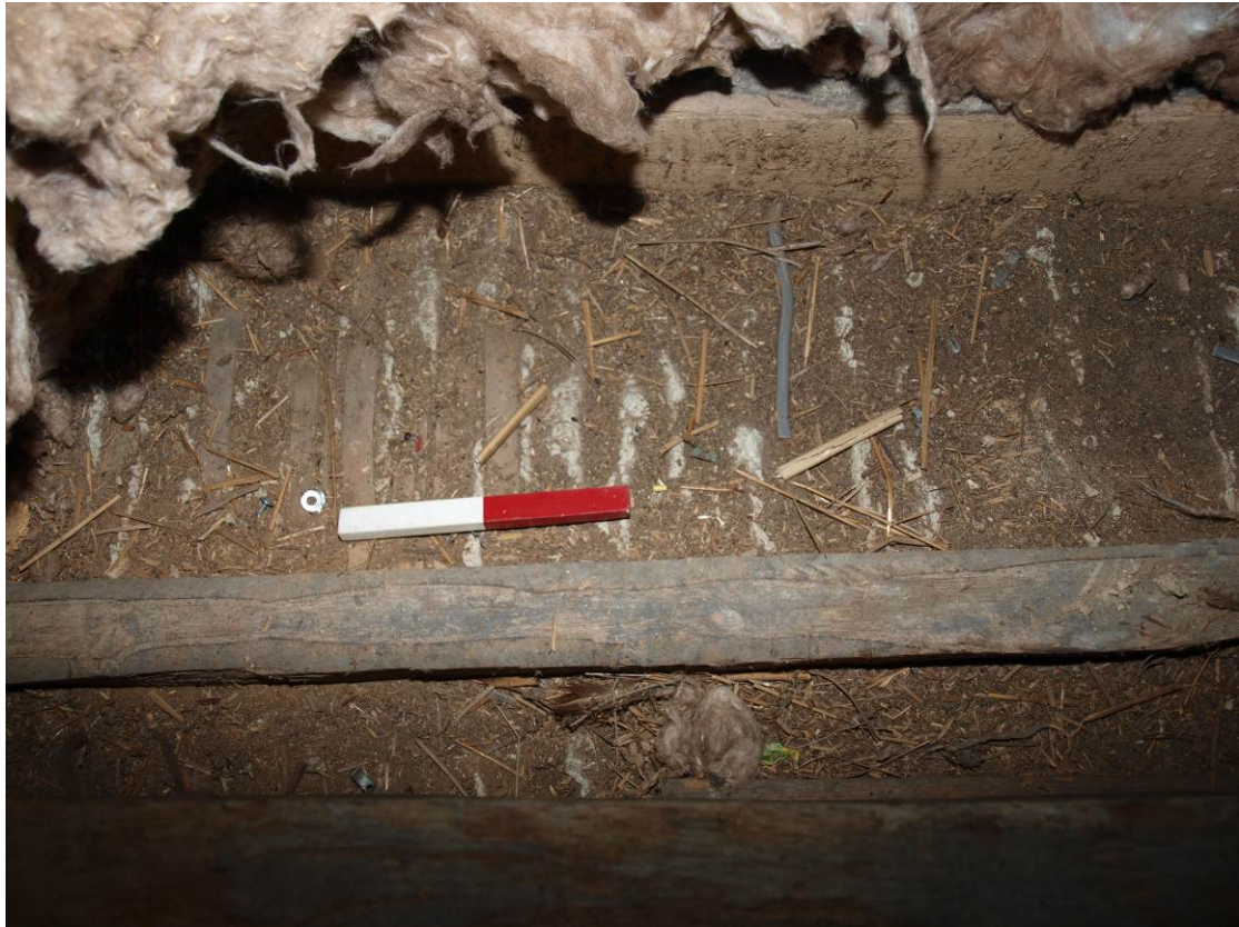
Plate 7: ?19 th century lath and plaster ceiling (20 cm scale)
