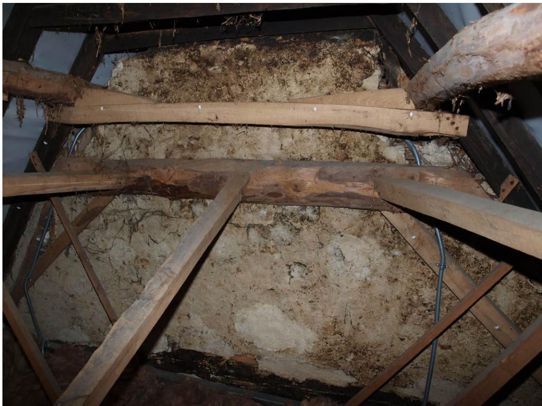
Plate 4: Lime skimmed T2 truss partition between hall and high end rooms
