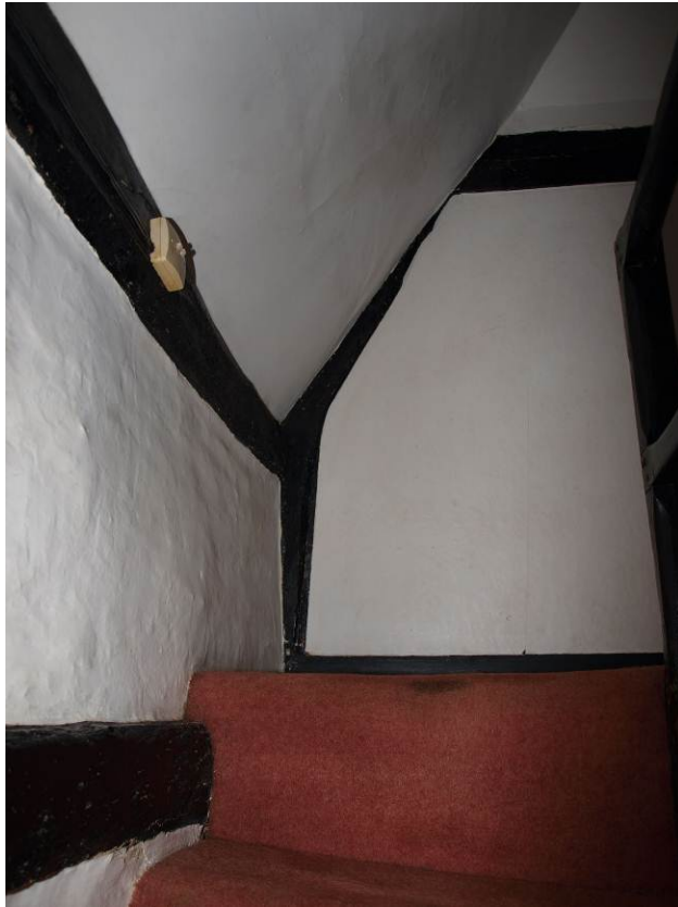
Plate 3: Cranked principal post (west side)
