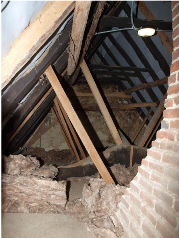
Plate 5: The cranked tie-beam of the T3 truss
